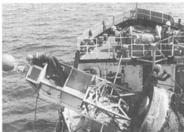
COMPLETING A LIGHTED SERVICE
